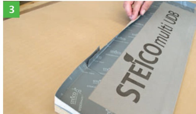
3 The STEICOmuli tape F adhesive strips are then attached to the insulation wedge in such a way that a three-sided „trough“ is formed.
