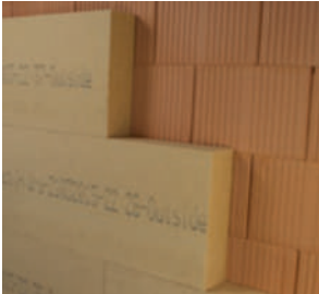
Installation of small-format square edge boards
