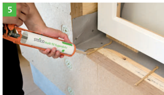
5 STEICOmuli fill adhesive beads are used to secure the insulation wedge against lifting off, e \leq 30\text{cm} .
