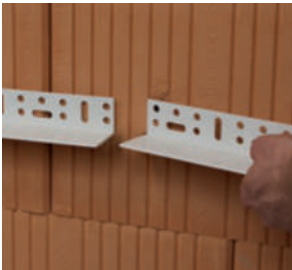
Attach angle rail
