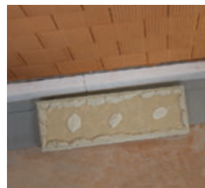
Adhesion of insulation boards on uneven surfaces using the point and bead method
