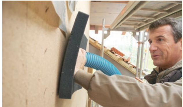
Air-injection hose in use with sealing sponge
