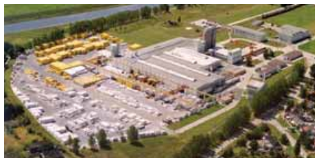
Calbe Factory, Germany
